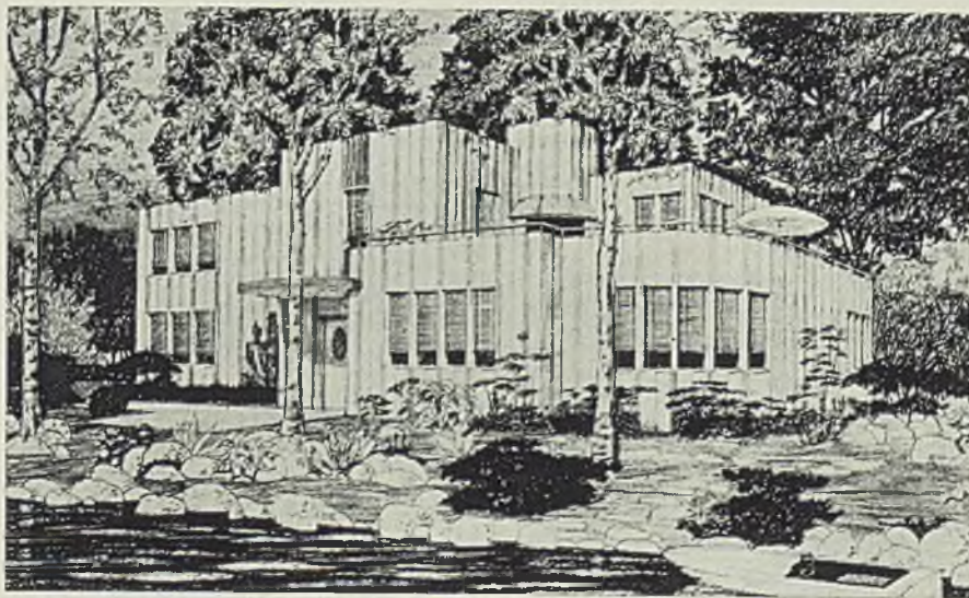
Structural steel framing and zinc exterior panels are features of this nine-room home being erected at Culver, Ind., for Dr. O. E. Bransky, Standard Oil Co. official
