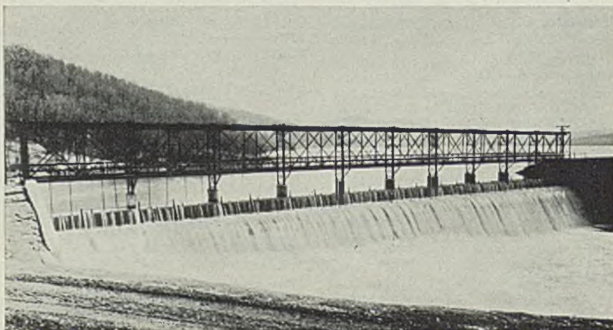
This is the famous Quemahoning dam at Johnstown, Pa., which held during the recent flood, under the most severe conditions in its history. The dam is 950 feet long on the crest, 20 feet thick at the top, and 700 feet in greatest thickness at the base. A new concrete spillway, 250 feet wide and 13 feet deep, was built by Bethlehem Steel Co. in 1933. The safety valve effect of this spillway was a helpful feature in the protection of the dam during the recent crisis
