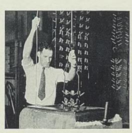
KOROLAC—new Goodrich discovery for coating plating racks—already has remarkable savings to its credit. For example, in the plant of a large automotive accessory maker, Korolac racks were tried in nickel and chrome-plating. Electric current consumption was reduced 40% and production so increased that a requisition for a generator (needed for increasing volume) was cancelled.
