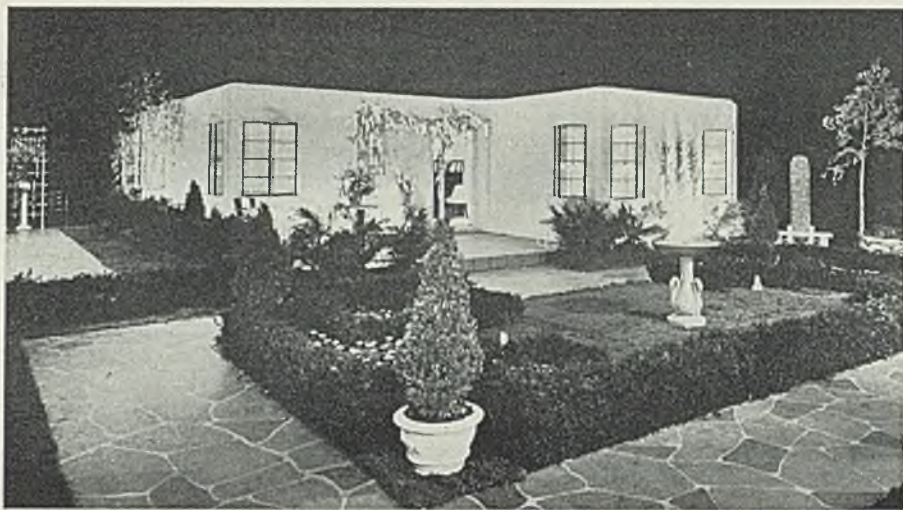
Displaying all-steel bungalows in department stores is the method adopted by one housing company for reaching prospective buyers. A house of the type shown above, completely furnished, drew an average of 2500 visitors a day in a Cleveland store recently
