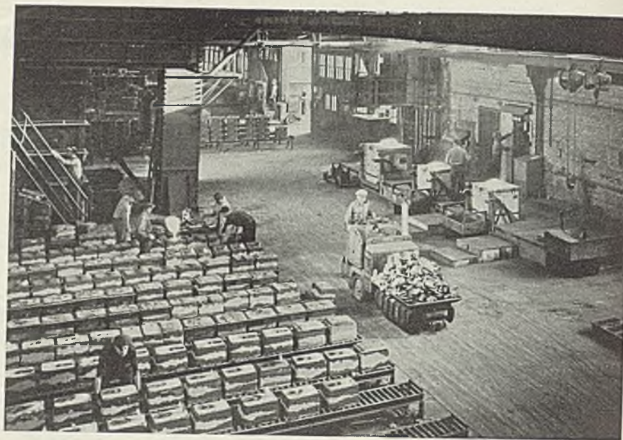
Fig. 2—Row of three induction melting furnaces and part of molding floor for handling small steel castings
