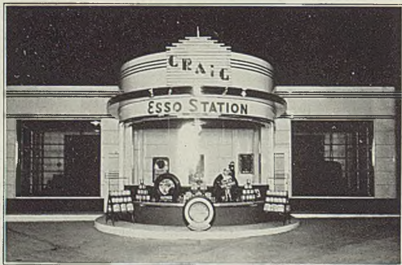
■ Porcelain enameled steel sheet in a red and white color scheme is featured on the front of Craig Service Station, Erie, Pa. Station is 26 x 48 feet and was designed and built by Erie Enameling Co., Erie, Pa. Illustration courtesy "The Ceramic Forum," 209 Fourth avenue, Pittsburgh
