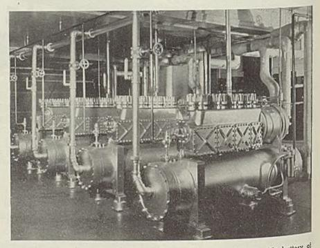
Air conditioning operating costs were reduced 40 per cent by this battery of four 40-ton Westinghouse hermetically-sealed condensing units, installed at State Lake theater, Chicago, by Kroeschell Engineering Co., Chicago. Units are automatically controlled, use suction gas to cool the driving motor. They require only one-fifth the floor space used by the 15-year-old, less powerful plant they replaced
