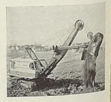
making adjustments easily and quickly. Ratchet type chocking brakes provide quick free move-up for either dragline or shovel, with automatic locking against the pushback of the digging action. For dragline work on soft ground, extralarge tapered "swamp cats" are available.
