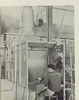
by a combination mercury-Mazda lighting system. Each of the mercury-Mazda units contains 400 watts of mercury lamps and 450 watts of Mazda lamps to provide balanced lighting. Spaced on 20-foot centers throughout the working area, these fixtures afford ample illumination for the most critical work and help assure quality in the finishing department.
