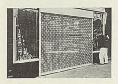
through the perforated ears of the links and forming the hinges. This allows structure to coil closely overhead around a horizontal pipe shaft which contains the counterbalancing springs.
