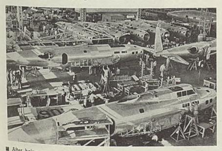
After being assembled in a series of steel jigs in another section of Boeing Aircraft Co's plant at Seattle, these B-17B bomber bodies take their place at the start of final assembly line. As each body receives its wings, on which landing gear has already been installed, it is rolled forward in the line. Body in middle of picture is just being lowered by overhead cranes to its place on assembly floor British, French To Co-ordinate War Buying
