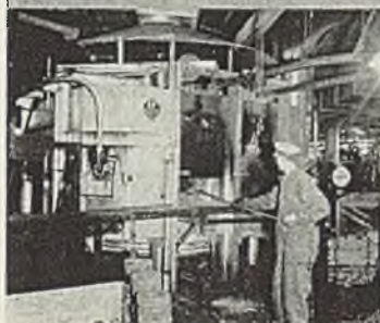
An E.F. Fuel Fired Rotary Furnace—used for normalizing and hardening—in the Wright Aeronautical Corp. plant.
