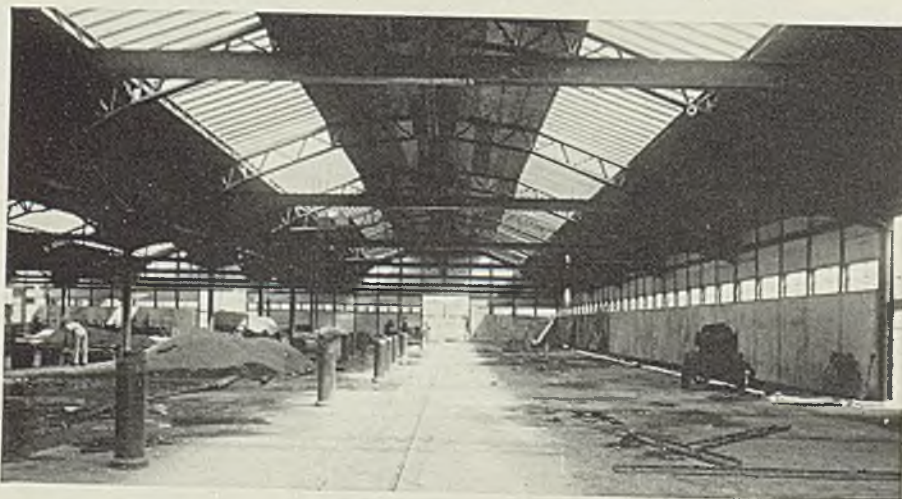
Fig. 2—General view of finished factory bay, one of five 60 x 240-foot bays forming complete building. Note large uninterrupted floor area and abundance of natural light
