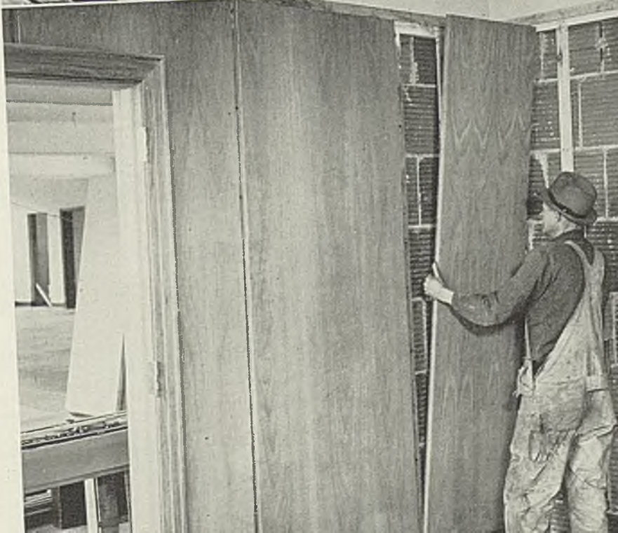
Fig. 6—Placing composite steel and wood veneer panels to form interior wall surfaces
