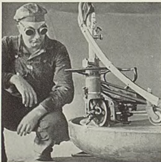
Fig. 2—Cutting an outside bevel on a dished head
