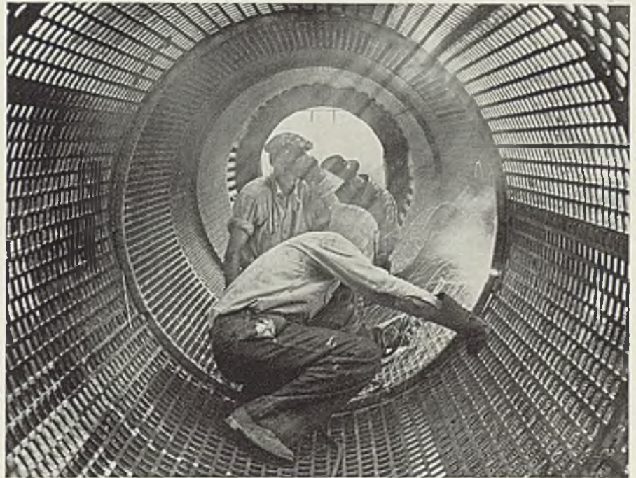
■ Shasta dam, second only to Boulder dam in height and exceeded only by Grand Coulee in mass, has made necessary the relocation of the Southern Pacific railroad along the Sacramento river in California. Preliminary work on the relocation project has been started at Pollock, Calif. To speed construction, these gravel screens are welded. Photo. courtesy General Electric Co., Schenectady, N. Y.
