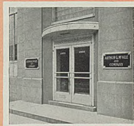
Entrance of the new McKee Building at 2300 Chester Avenue, Cleveland, Ohio.
