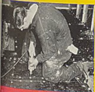
Man drilling holes preparatory to inserting and driving Thread-Cutting Screw.
