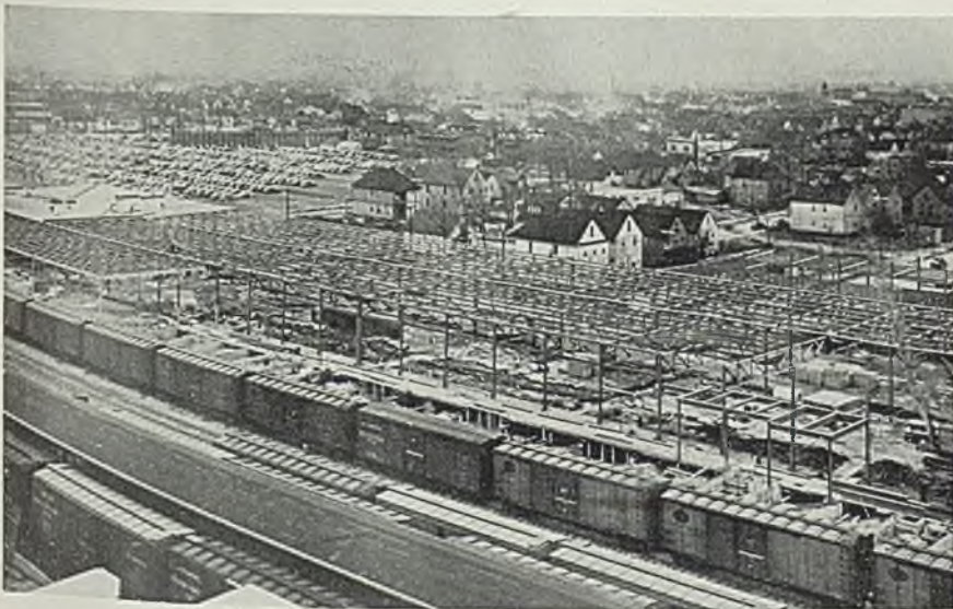
■ Front diagonal view of Packard's Rolls-Royce main assembly plant. Occupying a square block, this structure will house metallurgical laboratories, engineering laboratories, administrative staff and main engine assembly department. It is about two-thirds complete.
