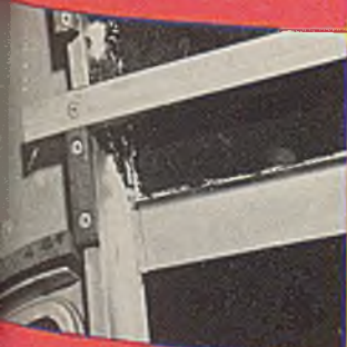
Section of wooden slats and railing atop metal frame of bus body.
