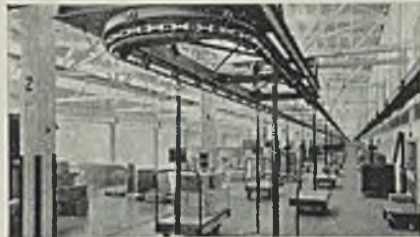
Link-Belt Overhead Conveyor moves the trucks automatically between stock rooms and shipping platform at the new warehouse of the Zellerbach Paper Company, Los Angeles. This system saves valuable floor space, since the conveyor is suspended entirely from the roof trusses.
