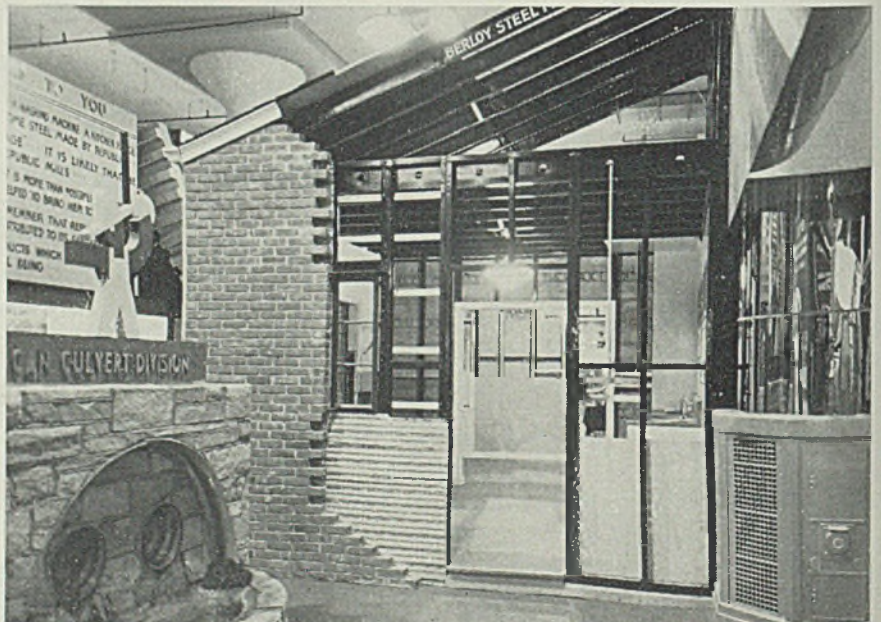
Adaptability of steel house frames to all types of exterior and interior treatment, various methods of insulation and a variety of designs are demonstrated in the open sections of the steel house exhibited by the Republic Steel Corp., Cleveland. The house is a product of the company's subsidiary, the Berger Mfg. Co., Canton, O.
