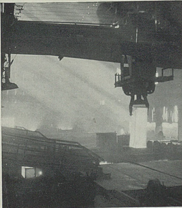
SYMBOLICAL of returning prosperity in the steel industry is the photograph taken in the Indiana Harbor, Ind., plant of Inland Steel Co., prosaically labeled "removing an ingot from a soaking pit"
