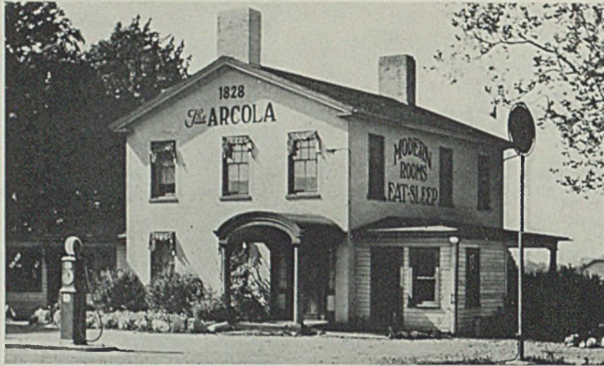
One hundred and eight years have wrought many changes in this old brick structure near Madison, O., once the headquarters of the Arcola blast furnace superintendent
