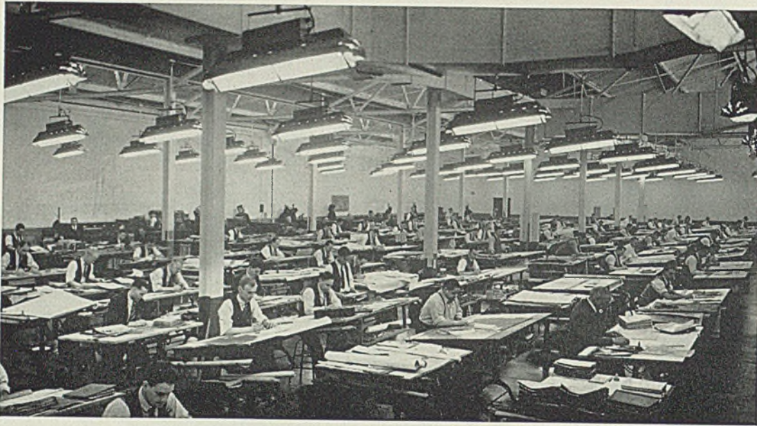
COLOR-CORRECTED light is provided in the drafting room of the International Harvester Co. by lighting fixtures combining mercury vapor and incandescent lamps supplementing skylights in the sawtooth roof. There are no windows
