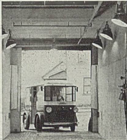
Center booth can be entered directly from street for the convenience of large trucks and trucks taken directly from service for refinishing
