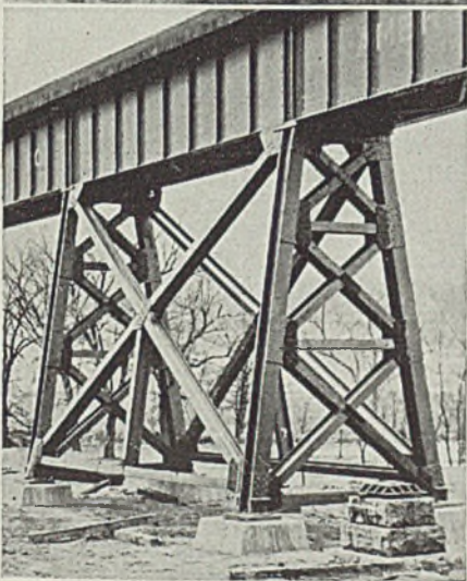
THIS single track, plate-girder viaduct was erected at Moravia, Iowa, by the Chicago, Milwaukee, St. Paul and Pacific Railroad Company. It was designed and constructed under the direction of their engineering department. Structural steel was fabricated by American Bridge Company.
