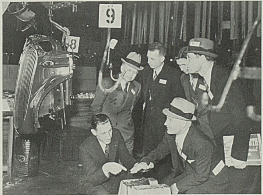
OTTO FRANKE (left), master mechanic at Plymouth Motor Corp., shows A.S.M.E. visitors to the Plymouth plant in Detroit how interruption of a light beam to a photoelectric cell stops one of the parts conveyors feeding the main assembly line. In operation, the part on the conveyor cuts off the light beam until it is removed to be placed on the chassis, thus preventing piling up of parts
