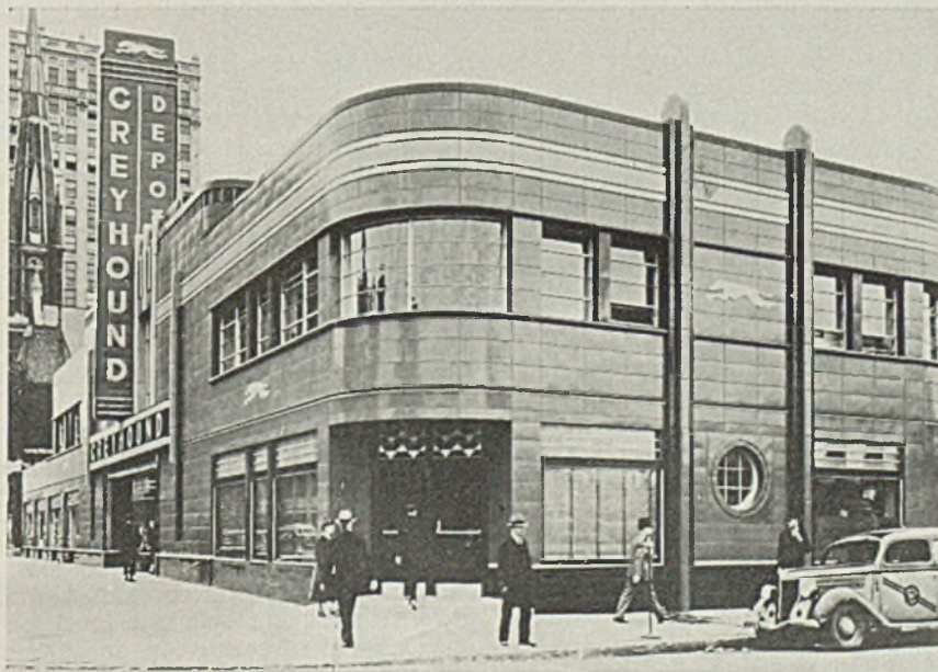
NEW Greyhound bus terminal, Louisville, Ky., shows effective exterior use of colorful porcelain enamels and decorative metal strips with glass brick. Grilles over doors and windows and balustrade for stairs inside are of white metal. Porcelain panels were furnished by Porcelain Metals Corp., Louisville, Ky., from enameling iron by American Rolling Mill Co., Middletown, O.
