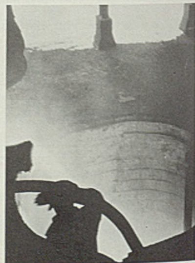
Fig. 2—Tapping a 100-ton heat of open-hearth steel
