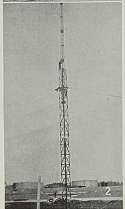
Fig. 1—Center tower has been erected and derrick mast is being raised into its regular position
