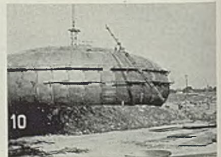
Fig. 9—Putting a side plate in place: The welded brackets are used here to support the scaffolding around the tank
