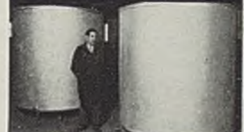
These Tanks for storage of Extracts were fabricated of Ingaclad by Sheet Metal Engineering Co., Chicago, Ill.
