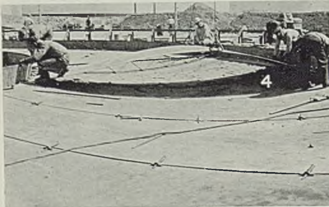
Fig. 7—Method of dead-ending ropes for plumbing the structure
