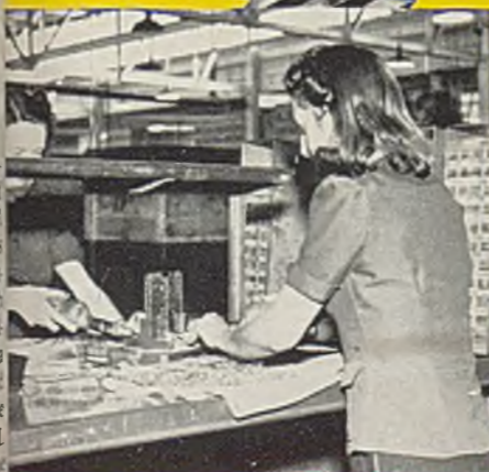
Girl operators making the important heating element and bus bar connections.
