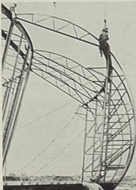
Fig. 11—Derrick mast is removed in sections
