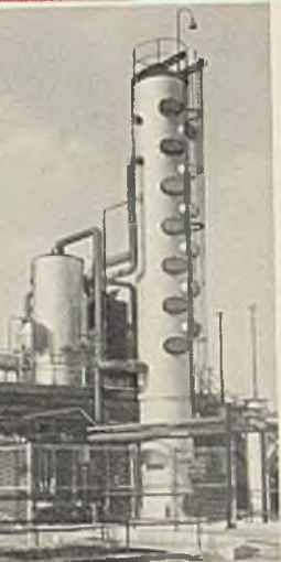
Light oil recovery plant at a mill has a capacity of 26,000,000 gallons of crude light oil per day, which is refined at an adjacent plant. There is a continuous wash oil purifier which removes muck from the circulating wash oil and prevents undesirable deposits in the scrubbed tubular equipment.
