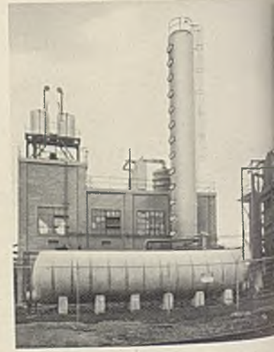
Koppers built the light oil recovery installation at this steel plant and a year later built a refining plant. It has a capacity of 10,000 gallons of crude light oil per day.
