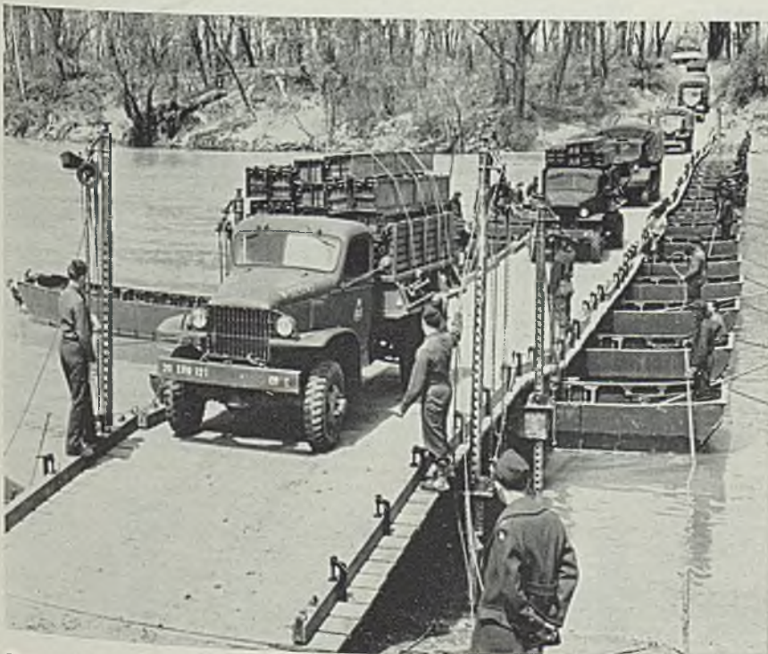
■ This pontoon bridge was thrown across the swift Chattahoochee river in 41½ minutes. In the foreground is a Chevrolet truck, assigned to the Army engineers, carrying a load of foot bridge units. The trucks also carry the bridge building equipment and tow the 10-ton pontoon boats on trailers
