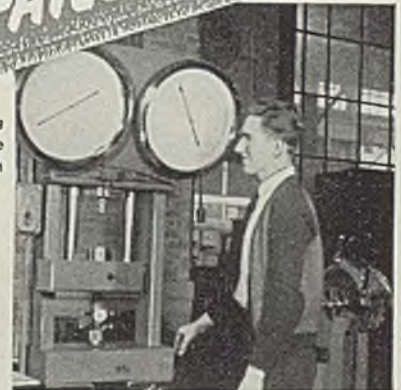
Testing to Determine Yield Strength
