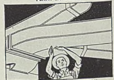
ALL KINDS OF DUCT WORK
