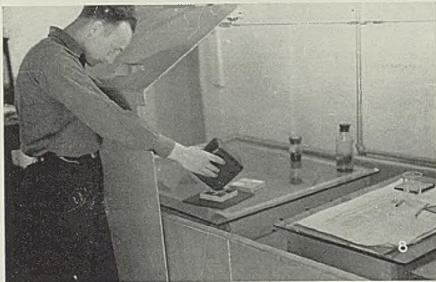
Fig. 7—Here fuzes have passed through many preliminary steps in assembly and are having their heads painted by dipping inverted into the paint. Note that fuzes are handled through assembly operations in racks of 25 units. In this portion of line, these racks are moved down the line between rails spaced the correct distance apart. Dipping is done by lowering a movable section of track over the paint tank. This station is also shown in immediate foreground of Fig. 2. After being inspected and set in racks in boxes, the fuzes are passed through the small opening in the wall into the
