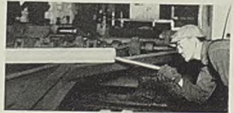
Each tube is inspected red hot, seconds after piercing.
