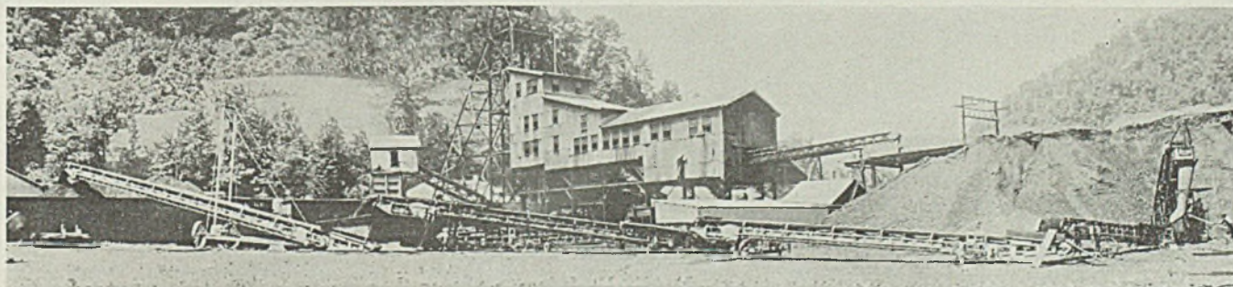
FIG. 1 (below)—Coal at captive mine is placed in storage by a string of portable conveyors which are mounted on high platform shown in background. Fig. 2 (right)—Coal being reloaded by mechanical loader and same group of portable conveyors used for storage
