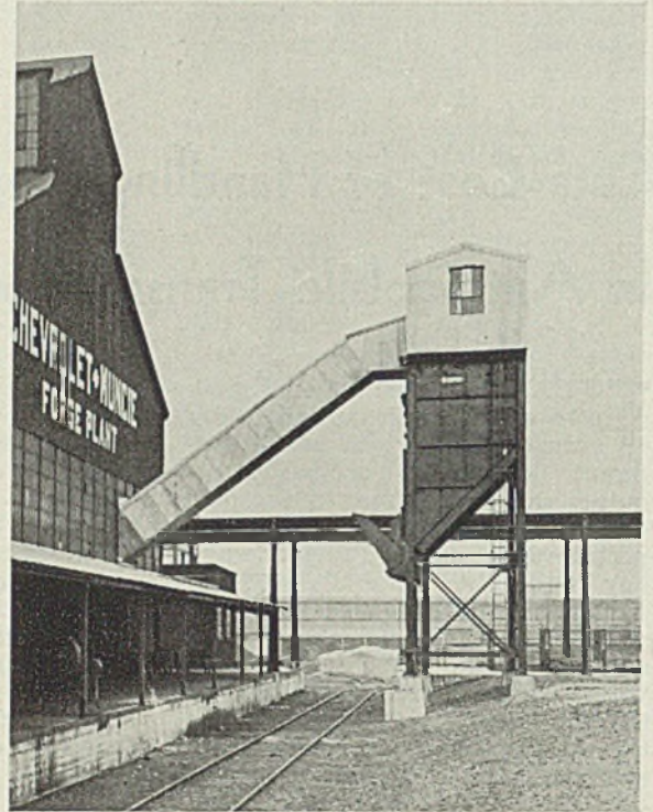
FIG. 4—Carried up this incline by the endless conveyor, the baskets dump their loads of flash in the proper bin and continue around for another load
