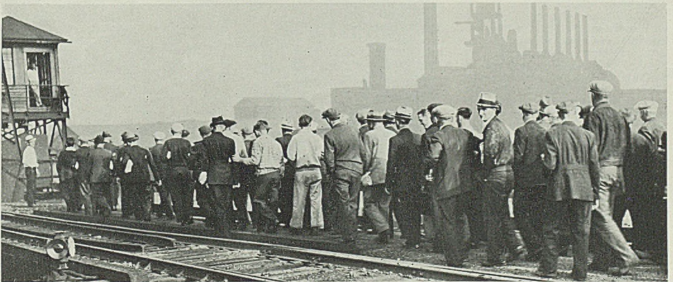
Given protection by state troops and police, a steady stream of steelworkers filed into Republic's Corrigan-McKinney plant, Cleveland. Three hundred had to be turned away Friday because the bar mill was not yet ready for operation. Open-hearth steel was poured for the first time in 44 days. Acme Photo
