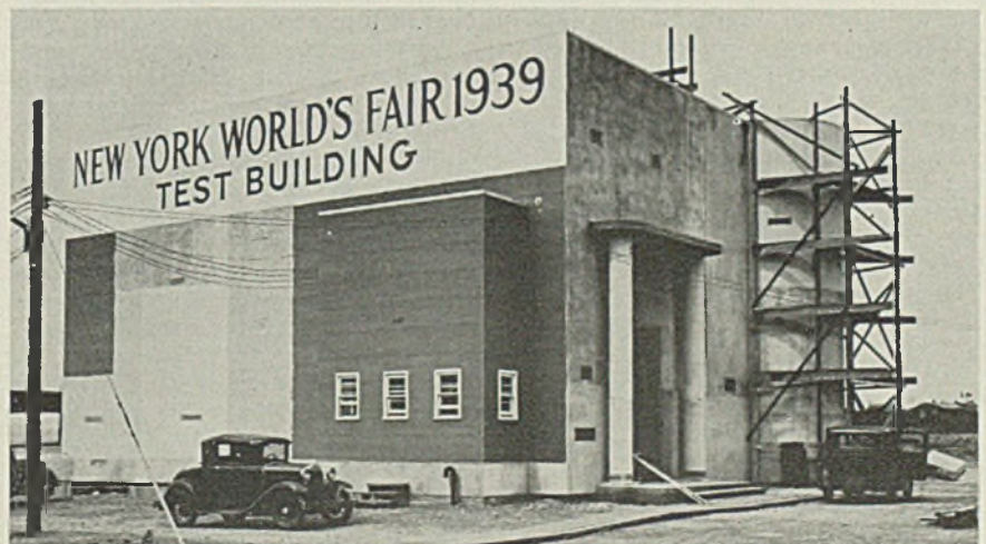
New York fair authorities are taking no chances on the materials which will go into many structures. The test building, with framework of steel, can reproduce all the twisting to which the buildings to be erected upon the filled-in Flushing Meadows, may be subjected
