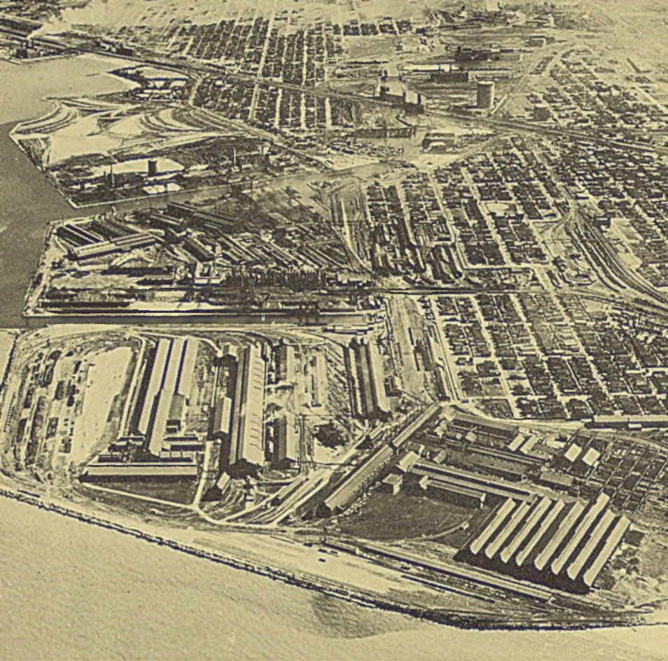
South works, Carnegie-Illinois Steel Corp., South Chicago, Ill.
