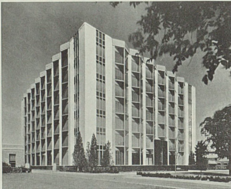
A. O. SMITH CORPORATION RESEARCH AND ENGINEERING BUILDING
