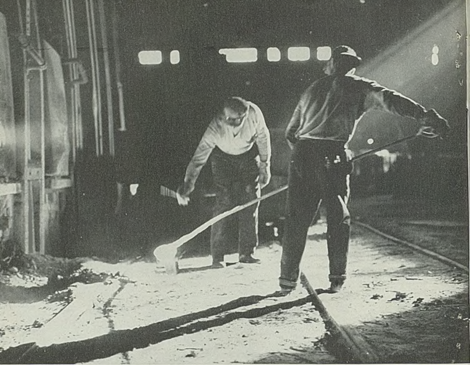
Pouring a Test Pig at an Inland Open Hearth
