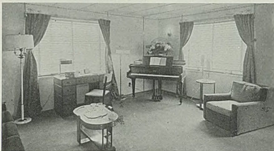
Interior surfaces of all steel homes lend themselves to artistic effects when given proper treatment, as reflected in this typical living room
