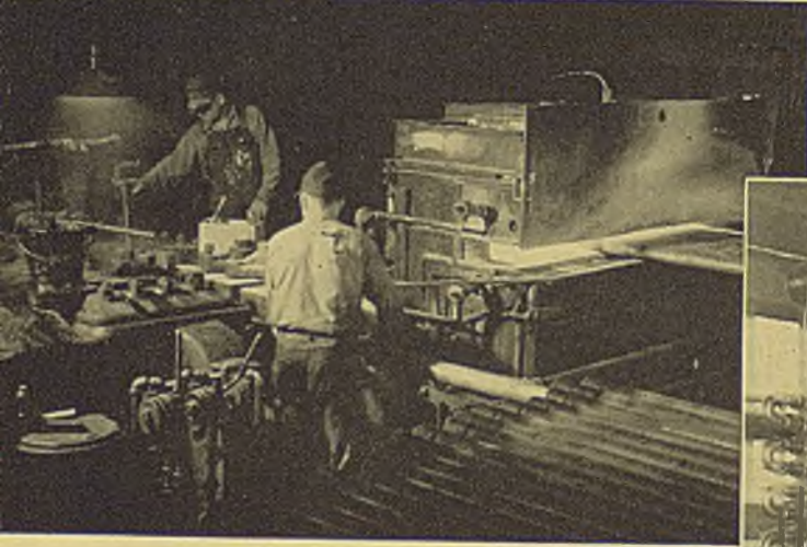
Above, upsetting ends of steel tubes while hot Below, this welded bed for record size press uses 11-inch plate and weighs 173,000 pounds
