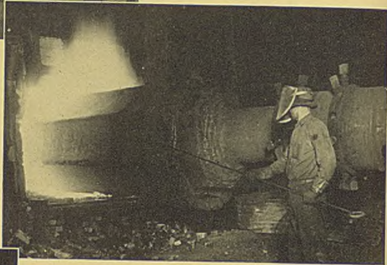
Below, welding a beer cooler for use in a large brewery
