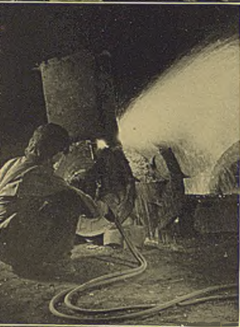
Above, condenser flanges being cut from steel plate
