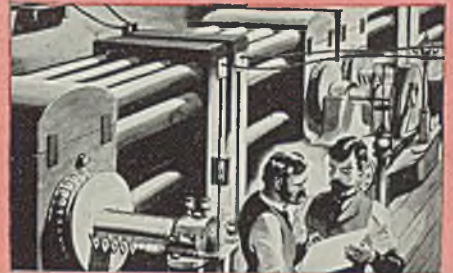
Man's dream of harnessing thunder-bolts was realized when in 1882 the first central station went into service. R B & W—then in business for 37 years—aided materially in developing electrical energy.
