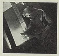
In marine work, Genex speeds work where lap welds are required on bulkheads and hull plating.
