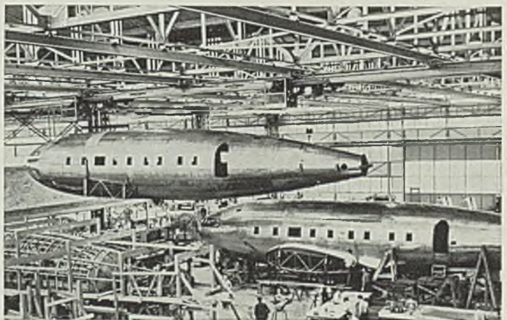
Two cabs operate on long span crane.
