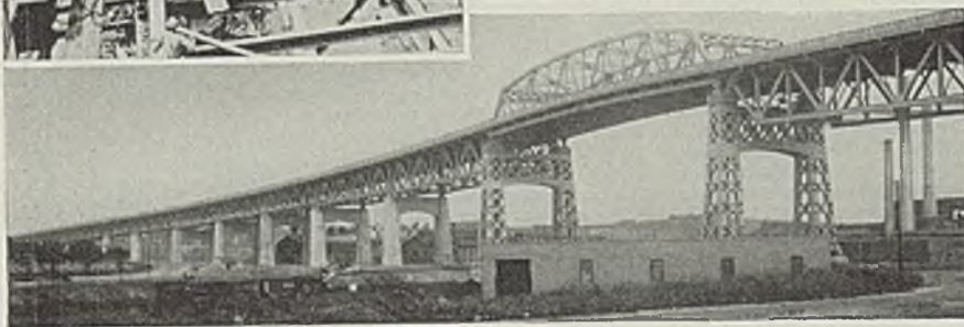
New York City's Meeker Avenue Bridge, most important link of the new Connecting Highway between the boroughs of Queens and Brooklyn, is 3500 feet long and carries two 32-foot roadways. Rising from grade, it overpasses existing streets and crosses Newtown Creek with a 120-foot navigation clearance.
