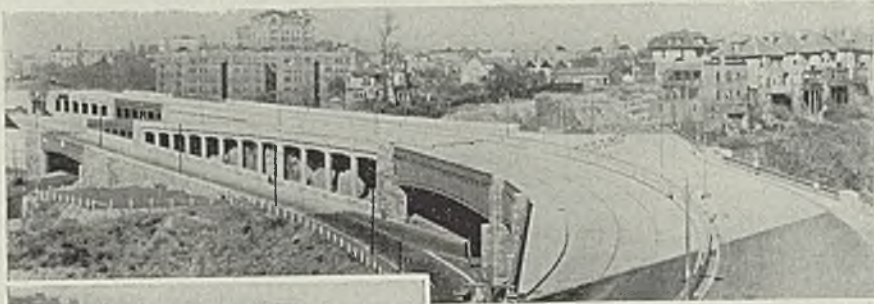
The deck plate girder overpass spans of the Lincoln Tunnel Approach at Weehawken, N. J., involved non-parallel alignment, skewed abutments, grades, curves and ramps. Ranking among the largest ever built, some of the plate girders erected on this project ranged up to 144 feet in length and 100 tons in weight.
