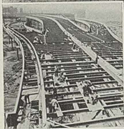
The deck plate girder overpass spans of the Lincoln Tunnel Approach at Weehawken, N. J., involved non-parallel alignment, skewed abutments, grades, curves and ramps. Ranking among the largest ever built, some of the plate girders erected on this project ranged up to 144 feet in length and 100 tons in weight.
