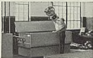
Vapor Cleaning Assembled Transmission.
