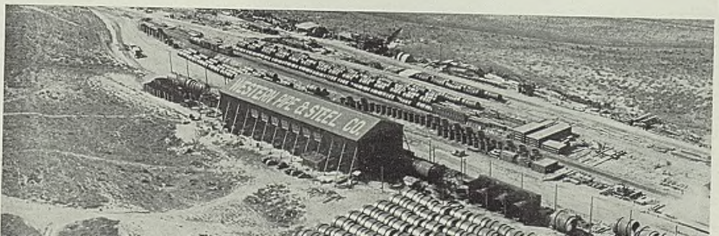
Fig. 1. (Bottom)—Plant erected especially for lining fabrication. Fig. 2. (Center)—Templet used in welding stiffener rings. Fig. 3. (Top)—Gantry crane handles lifting and moving in plant and at storage areas at each end. Photos courtesy American Chain & Cable Co., Bridgeport, Conn.
