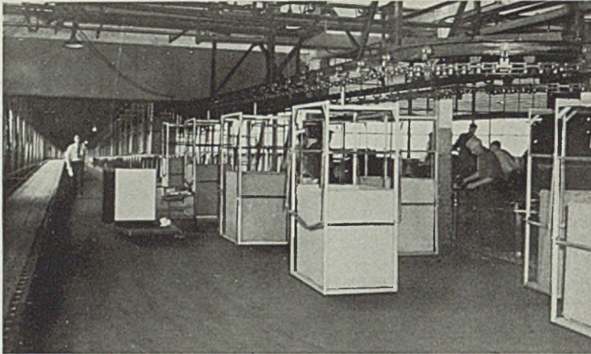
Fig. 2—Interior view showing reversible belt conveyor line at left, 6-foot aisle for trucks and continuous 2-way overhead chain conveyors at right
