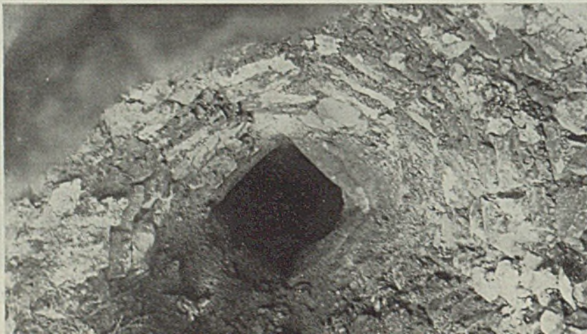
Fig. 2—View of furnace shaft looking down into the bosh and hearth
