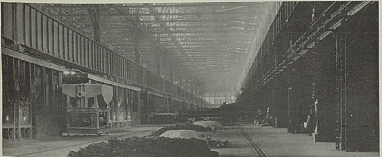
Battery of basic open-hearth furnaces with raw materials in foreground
