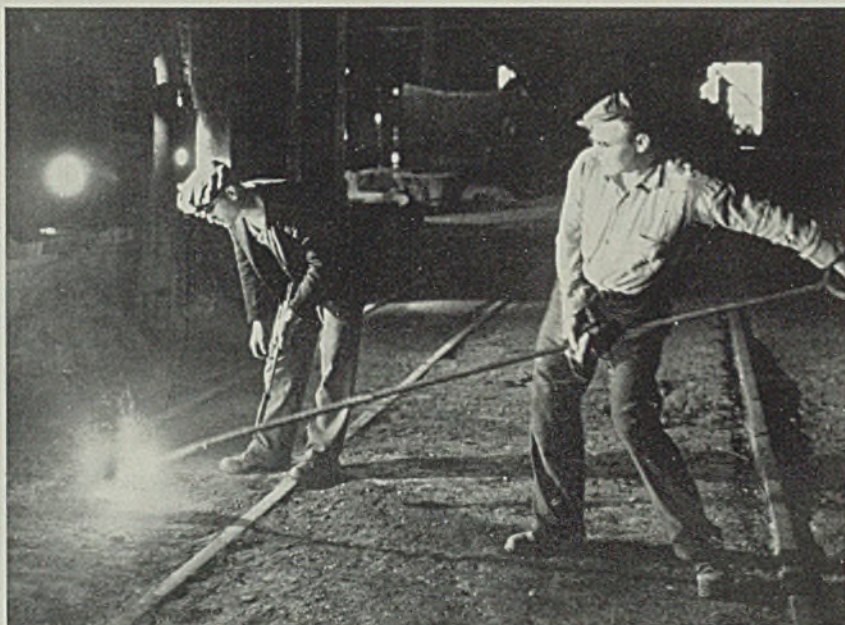
Taking a preliminary test sample of an open-hearth heat
