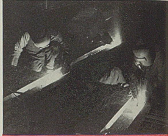
Fabrication by welding.
