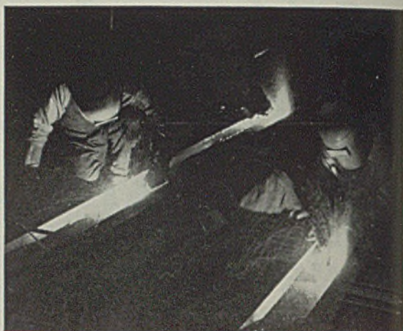
Fabrication by welding.
