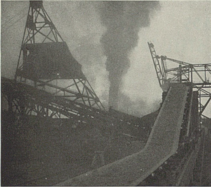
View of 470-foot dock conveyor with tripper mechanism causing discharge of ore to gantry at extreme right with gantry at any point along the dock conveyor. Illustrations courtesy Link-Belt Co., 307 North Michigan avenue, Chicago
