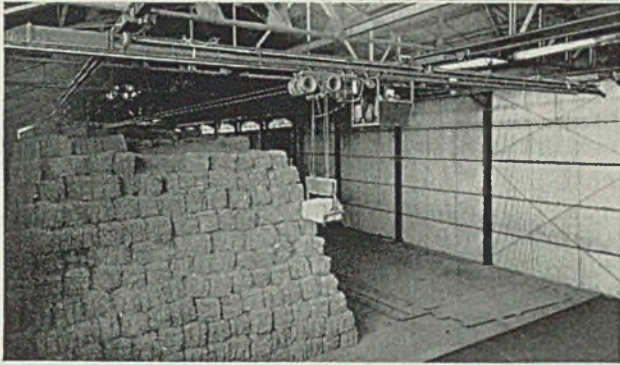
A single 1½ H. P. motor drives a 62 ft. crane.
