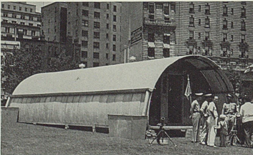
■ Corrugated steel tropic shelter which can be erected in nine hours is demonstrated by United States Marines at Washington. The hut can be covered with dirt or sandbags as camouflage and protection from shell splinters. NEA photo
