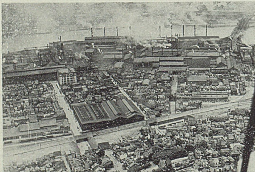
HOMESTEAD: Now undergoing a major geographical operation to make room for Carnegie-Illinois' new armor plate plant, this famous mill town soon will present a radically changed appearance. NEA photo
