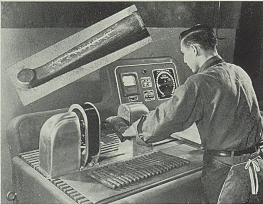
■ In inspecting all parts important to the safety of the driver, Studebaker's South Bend plants make use of the above Magnaflux which shows up defects not discernible with a 100-power microscope. Parts are first magnetized by the unit and then sprayed with ferromagnetic powder which adheres to the imperfection. Note the part inset above
