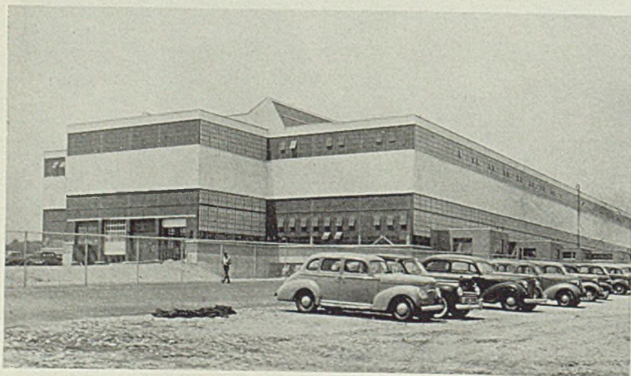
■ New machine tool assembly building of Bullard Co., Bridgeport, Conn., is largest of several additions built by the company during the past year to meet expanding defense requirements
