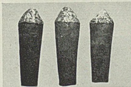
Below: Tang bits made of .60-70 carbon steel with a semi high-speed steel core as a wearing surface last approximately one hour. Those faced with Stoodite give up to 20 hours' service without need for redressing.
