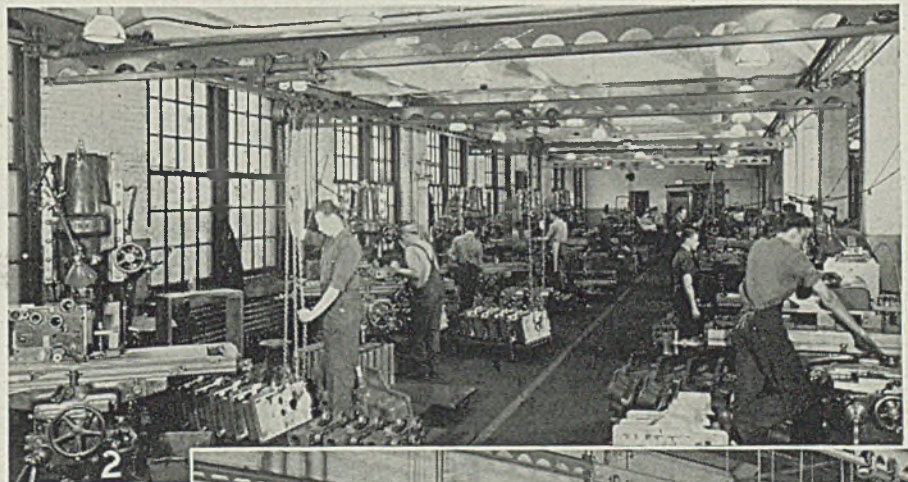
Fig. 2—A battery of hand-operated tramrail cranes in the heavy duty vertical milling machine department at Warner & Swasey plant, Cleveland
