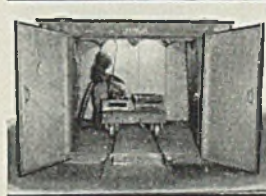
AIR BLAST ROOMS
