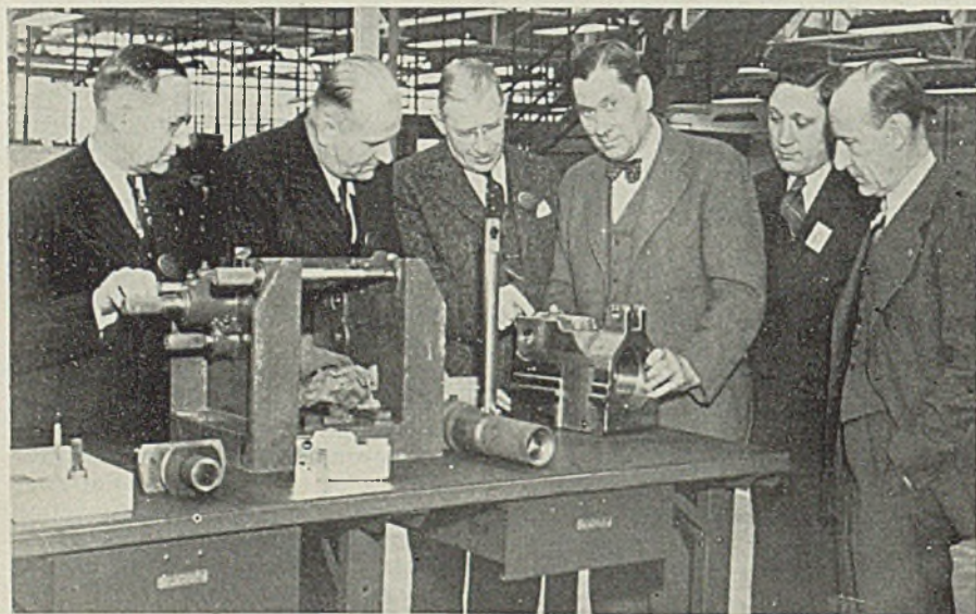
THREE months after the first structural steel was delivered. Chrysler Corp. started operations in an annex to one of its auto factories now devoted to war production. New building is operating 24 hours a day. Above, David A. Wallace, president, Chrysler sales division, is examining a breech ring produced in the plant. The part, weighing 310 pounds in the rough, is machined down to 105 pounds. Left to right: Charles Thiede, master mechanic; A. M. Fleming, general works manager; Edward H. Priebe, works manager; Mr. Wallace; A. P. Collies, superintendent; and Harry E. Watterson, plant engineer
