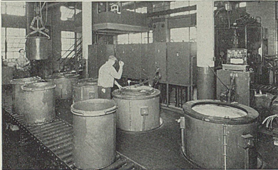
Fig. 4. (Bottom)—Pair of smaller rotary-retort units with their quench tanks and drying conveyors. Portion of loading conveyor chute can be seen at extreme upper left
