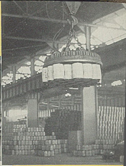
No. 6 Type SA Magnet handling kegs of Nails, Wire, etc., in warehouse. This lift consists of 29 kegs of 8-penny nails, 100 lbs. per keg.
